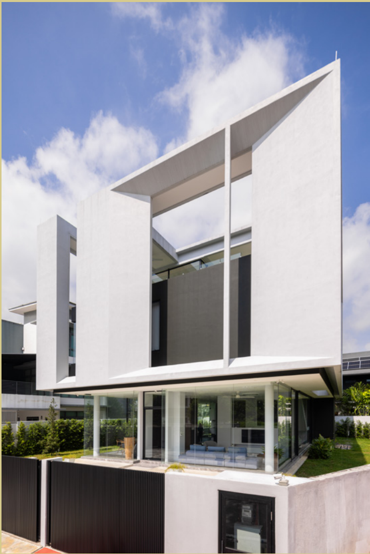
Reinforced concrete serves as the primary material, adding weight that accentuates the floating effect with a heavier mass at the top and a lighter form at the bottom
